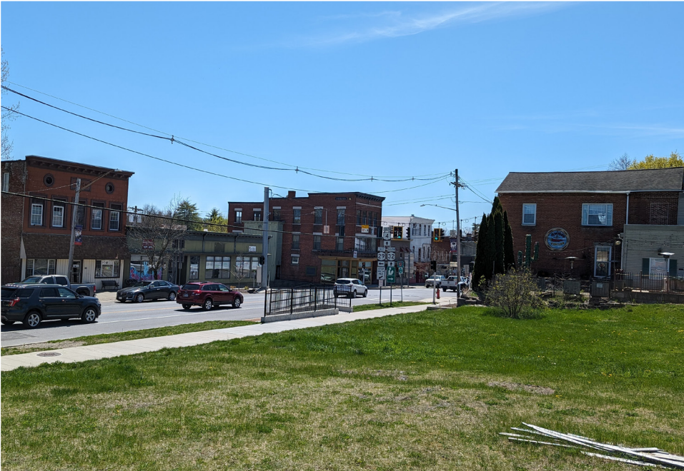
Above: Existing condition of the site
